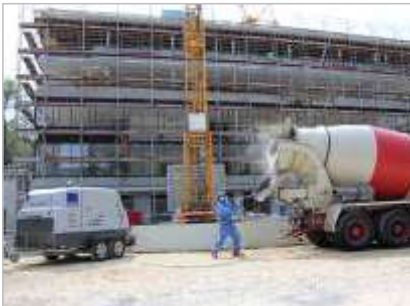
Ready Mix Concrete Truck Cleaning
