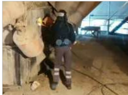
Pre Heaters Cleaning
