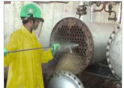
Power Plant Condenser Tube cleaning
