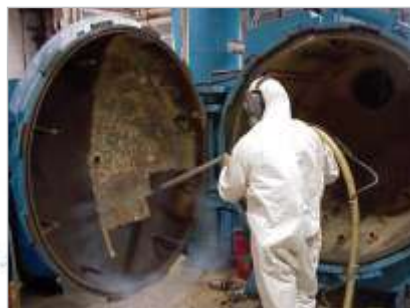
Cement Silo Cleaning
